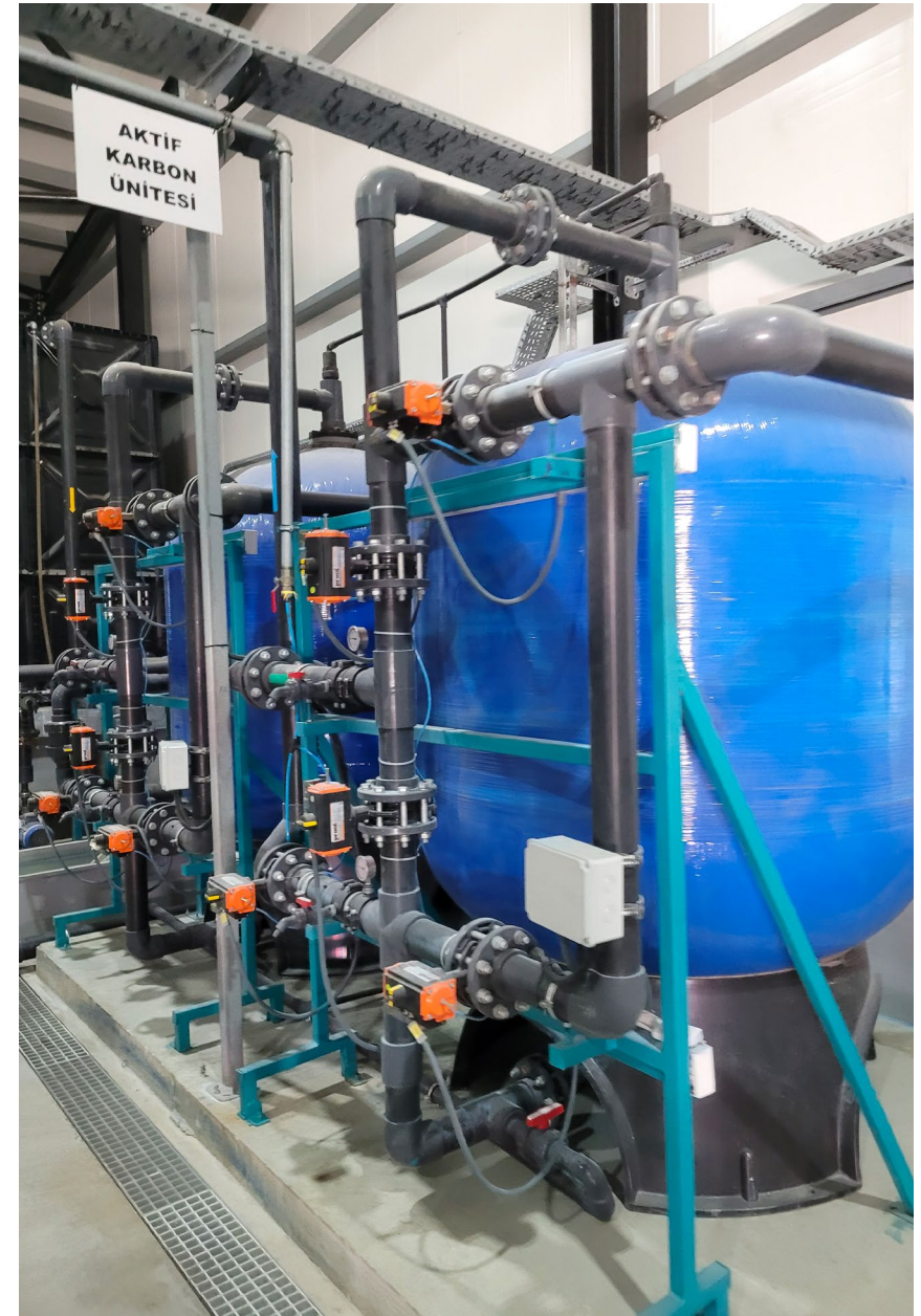
Carbon process for recycling water.
